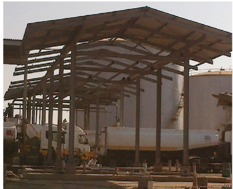
Gantry Works: Truck Loading Gantry Works
