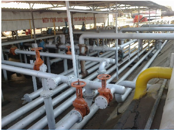
Pipe Linking: Fuel Pipe Connections & Fittings
