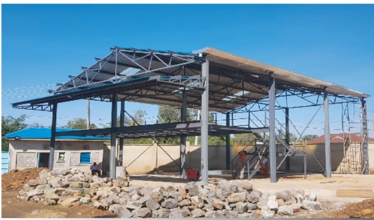
Warehouse with mezzanine floor
